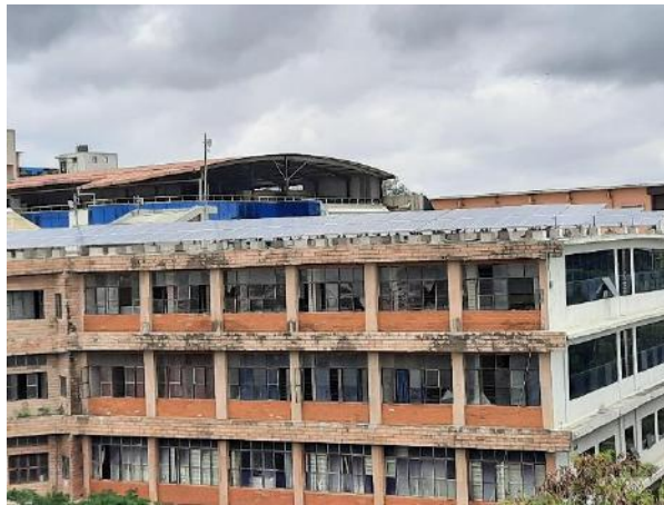
Photo 1.1 : Solar panels installed in MCA block
