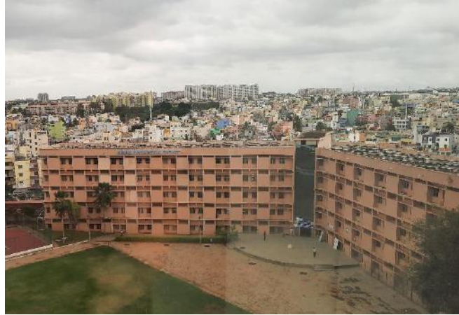
Photo 1.2: Solar panels installed in science block
